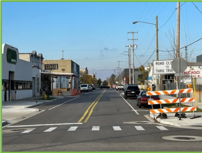
Ottawa Ave. Reconstruct in Grand Rapids; photo courtesy of GVMC Staff
