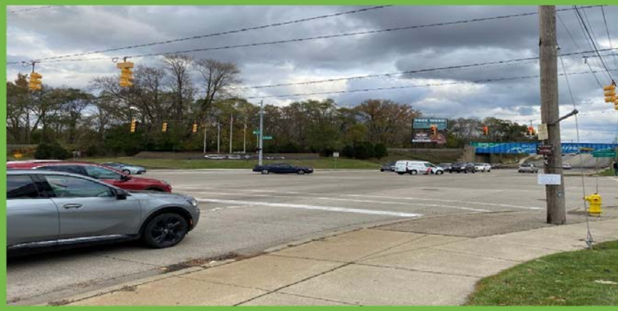
Intersection of 28th St. and Division Ave. S, which was ranked No.1 intersection for fatal and serious injury crashes from 2018 to 2022 in the GVMC area
