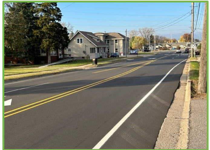
32nd Ave. Resurface in Hudsonville; photo courtesy of GVMC Staff
