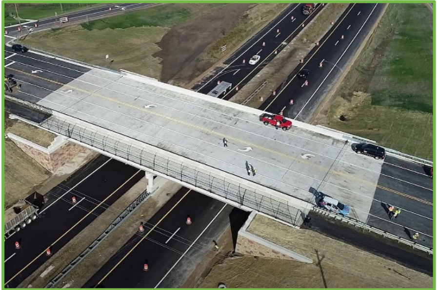
Picture of the completed 100th St. Bridge featuring active transport access; Photo Courtesy of MDOT
