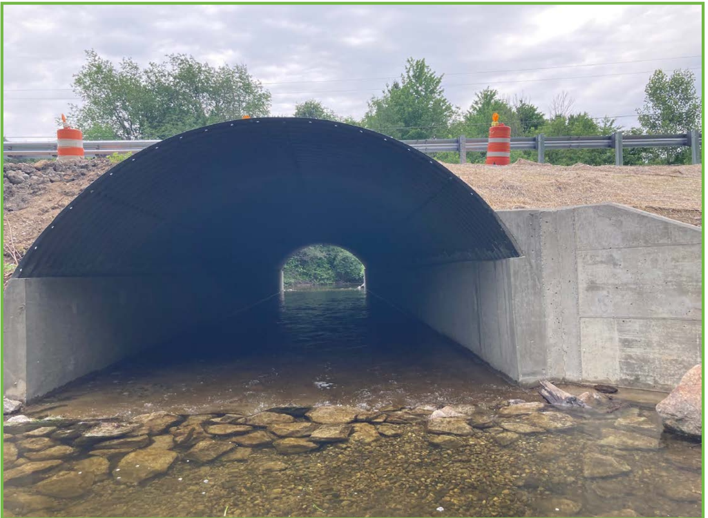
Bridge culvert rehabilitation project; photo courtesy of the KCRC
