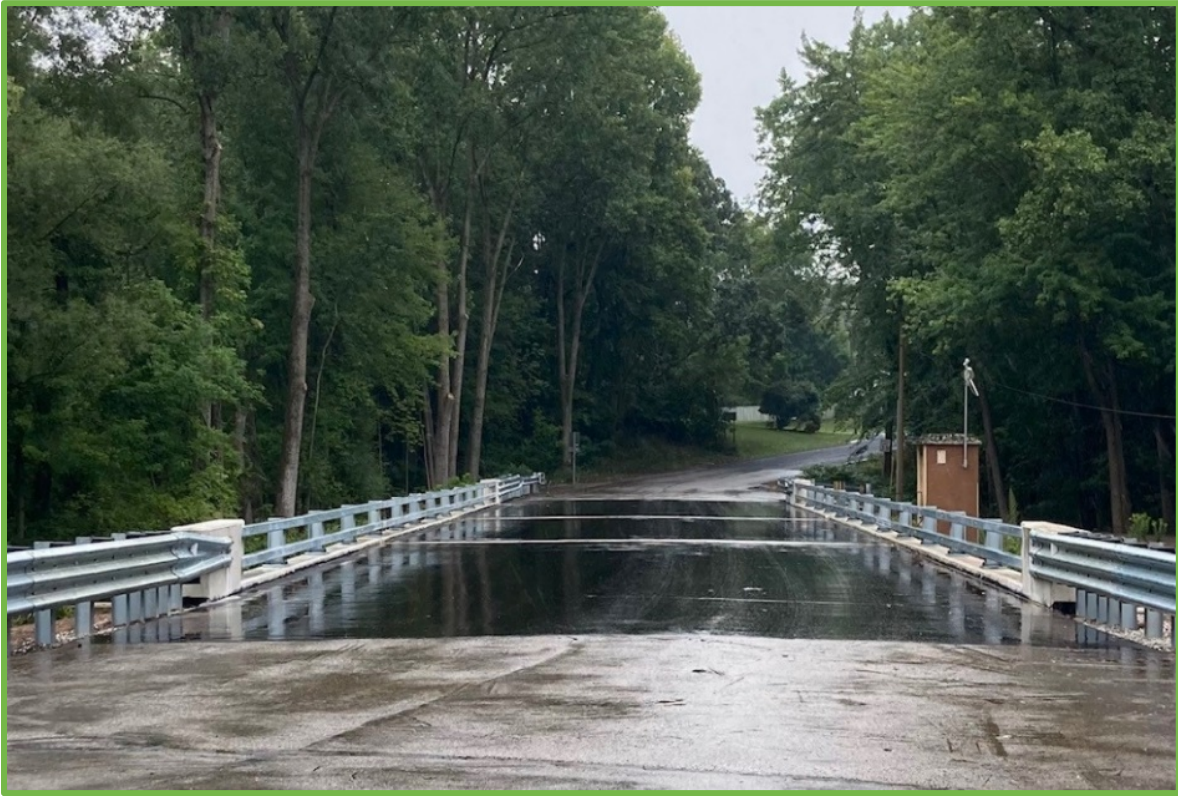
Packard Dr. Bridge over the Rogue River reconstructed this year in Plainfield Twp; Photo courtesy of Kent County Road Commission (KCRC)
