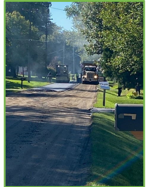
Resurfacing project in a Cascade Township neighborhood
