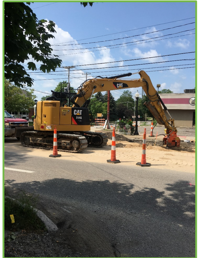
Construction project on E Fulton in Grand Rapids
